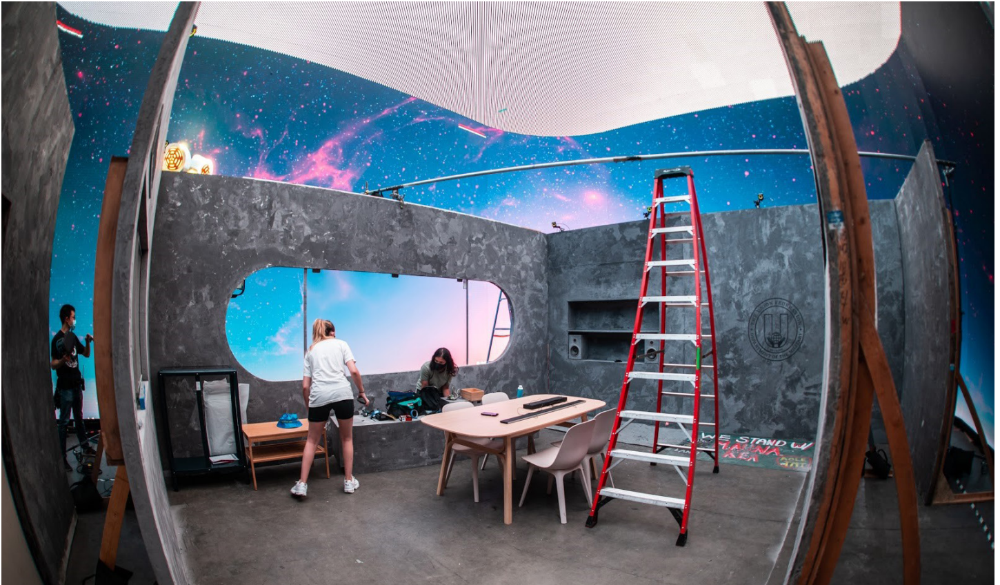
Dining Room Set construction
